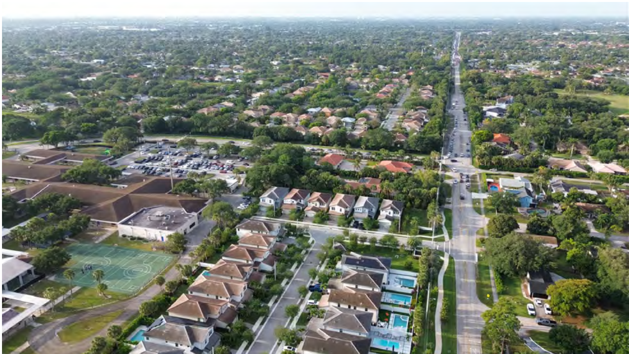
Figure 3-1: Barwick Road from Lake Ida Road to L-30 Canal
